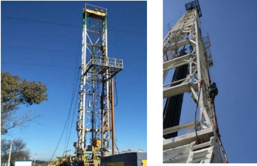
Figure 2: Mat de l'appareil forage rotary, BESAILET Abdelhak (2018)
